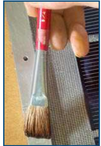
The tops of the sidebars are coated with silicone before placing the Plexiglas cover
